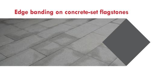
**Description:** Formation of cement staining resembling a picture frame around flagstones, visible a few days after installation.
