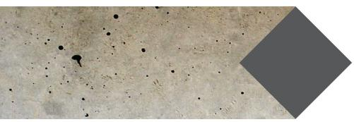
Description: Small holes that may appear on the surface of larger pavers during or after installation.
