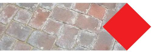
Description: White salt deposits that may appear on or near the surface of concrete, clay, and natural stone products.
